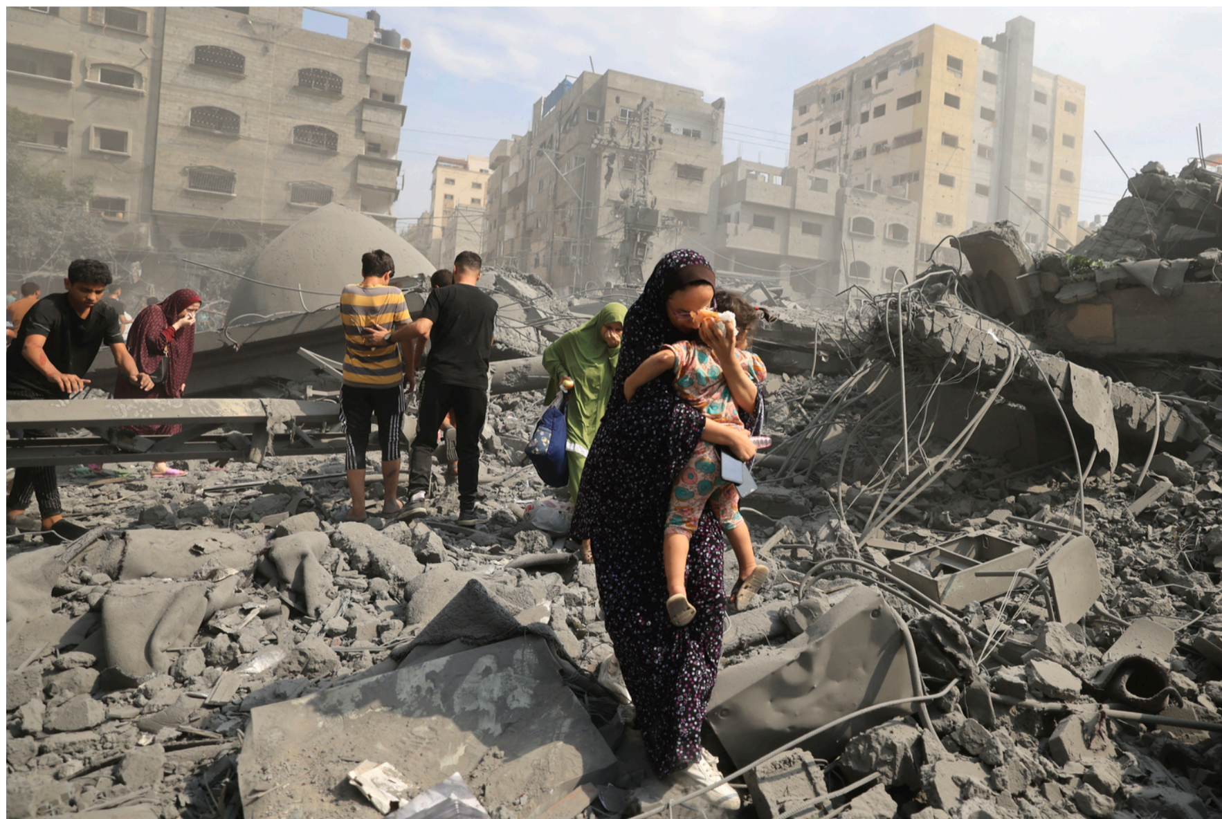
Palestinians in Gaza city inspect the damage following an Israeli airstrike, 9 October 2023, photo by Mahmud HAMS / AFP
