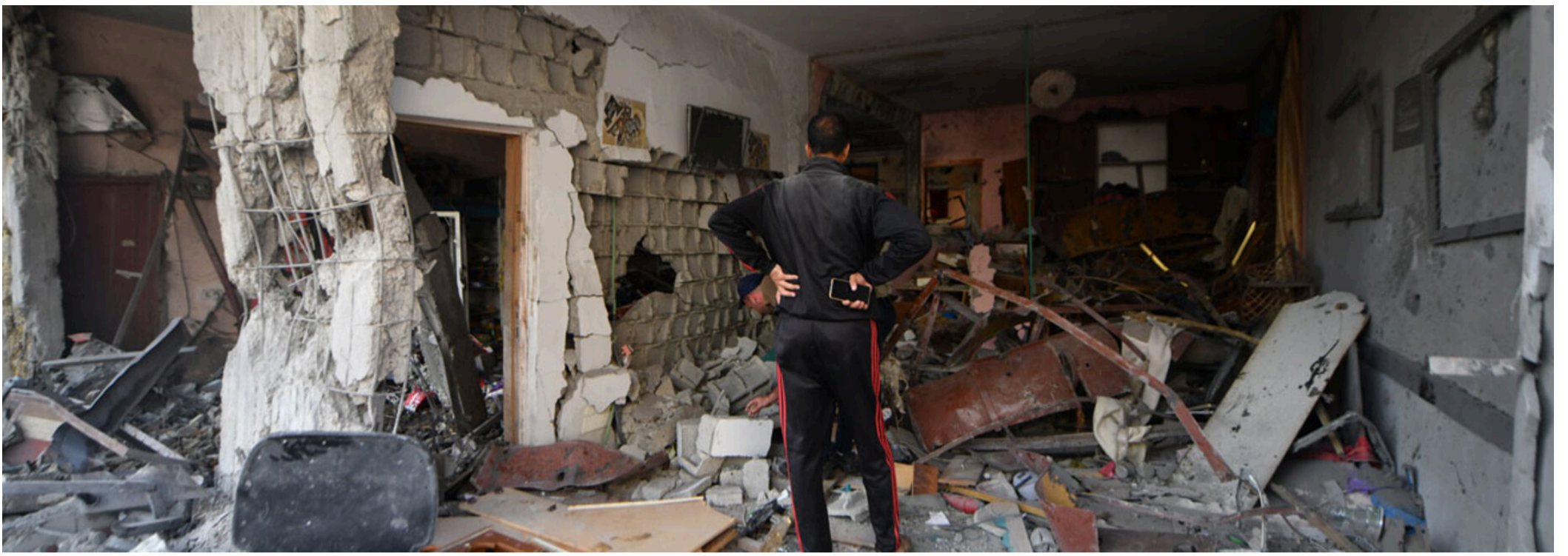
Jamal inspects his home in Khan Younis, in the southern Gaza Strip, after it was heavily damaged in hostilities. By 6 November, over 40,000 housing units across the Gaza Strip had been destroyed, according to the Ministry of Public Works and Housing. Photo by ©UNICEF/Zaqout, 16 November 2023
