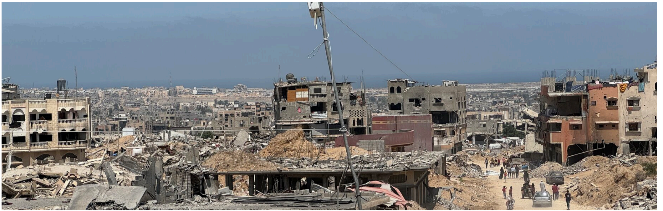
Extensive destruction in Bani Suheila, Khan Younis. UN teams reported that almost every building in the area was destroyed or damaged following repeated incursions. Photo: Themba Linden/OCHA
