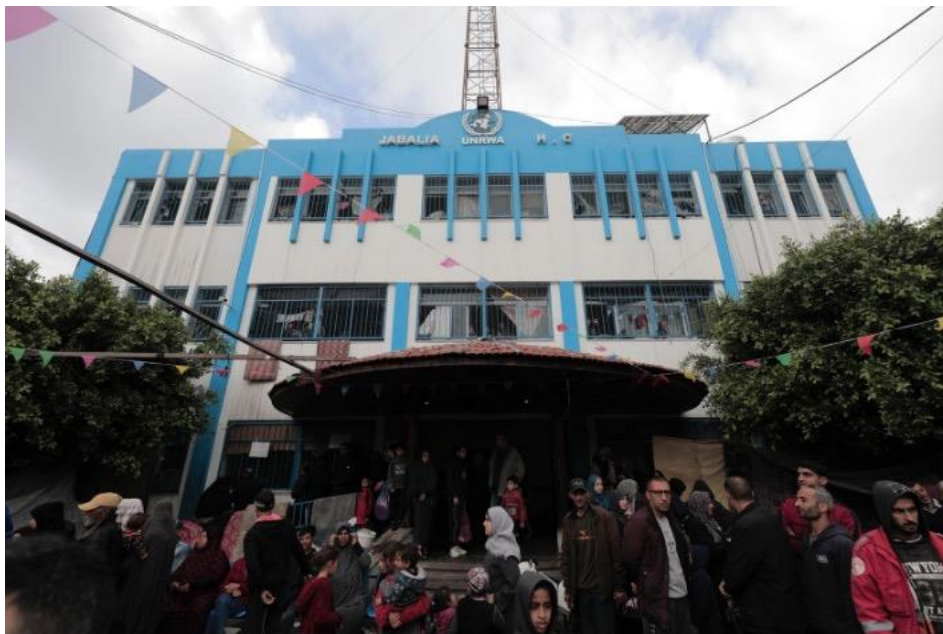
UNRWA Jabalia Health Centre before and after been hit. © 2024 UNRWA Photo
