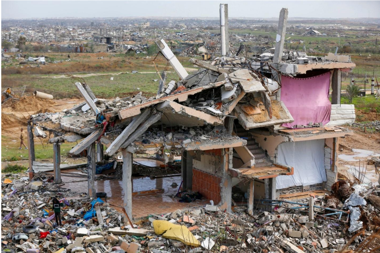
A destroyed house in Nuseirat, Gaza Middle Areas, February 2025. © 2025 UNRWA Photo by Ashraf Amra
